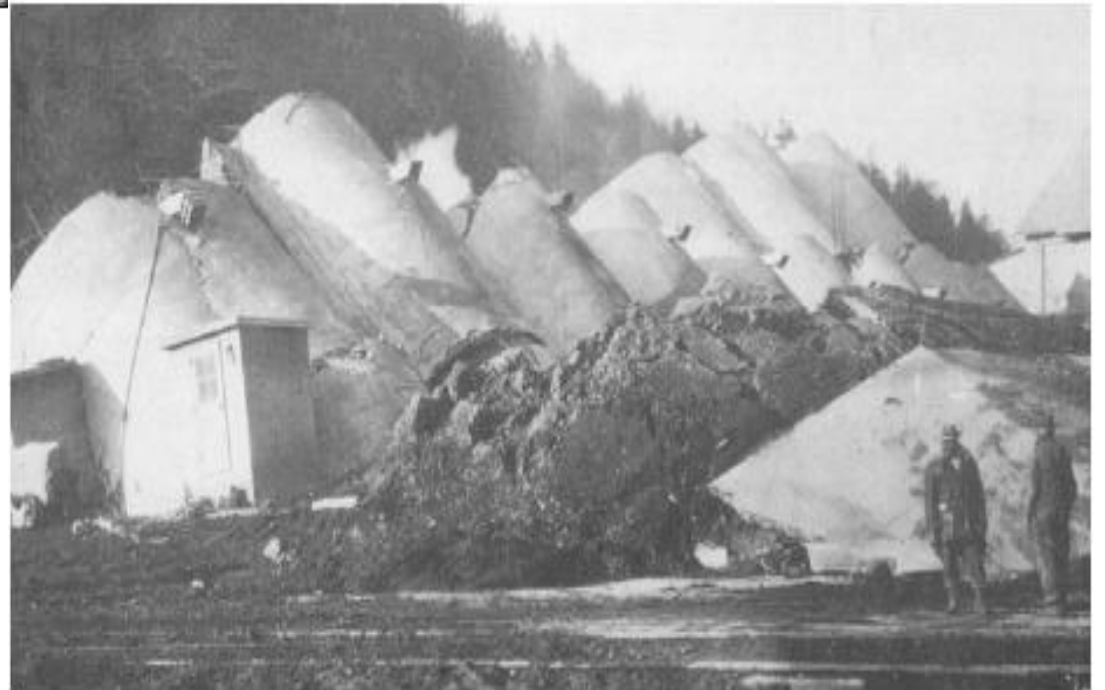
Figure 8-12. Bearing capacity failure of silo foundation (Tshebotarioff, 1951).
