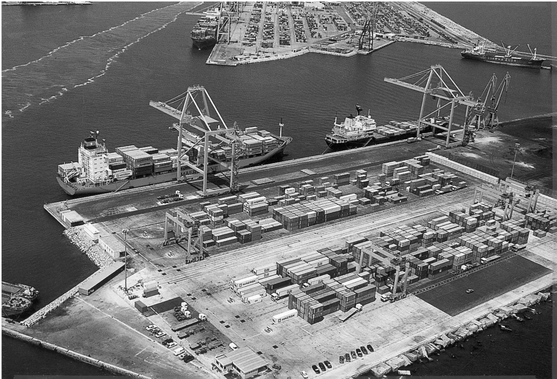
Figure 1.16 Container storage area; typical linear container stacking configuration.
